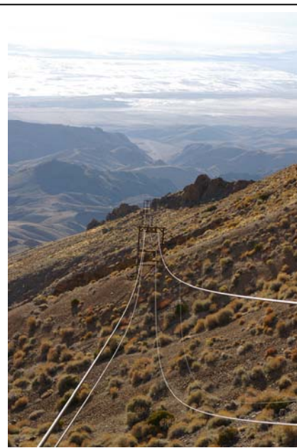
Looking down the wire-wrap cable of the Morning Star tramway, which ends at the Estelle tunnel. Circa 1906-1916. What a view.
