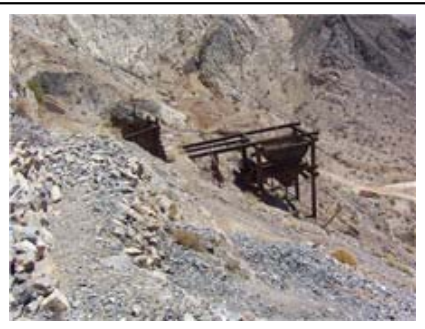
Mine dump chute at the Minietta Mine.
