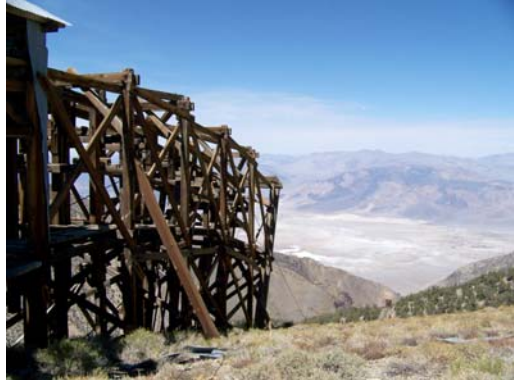
The Cross-over Tower looking down into Saline Valley.
